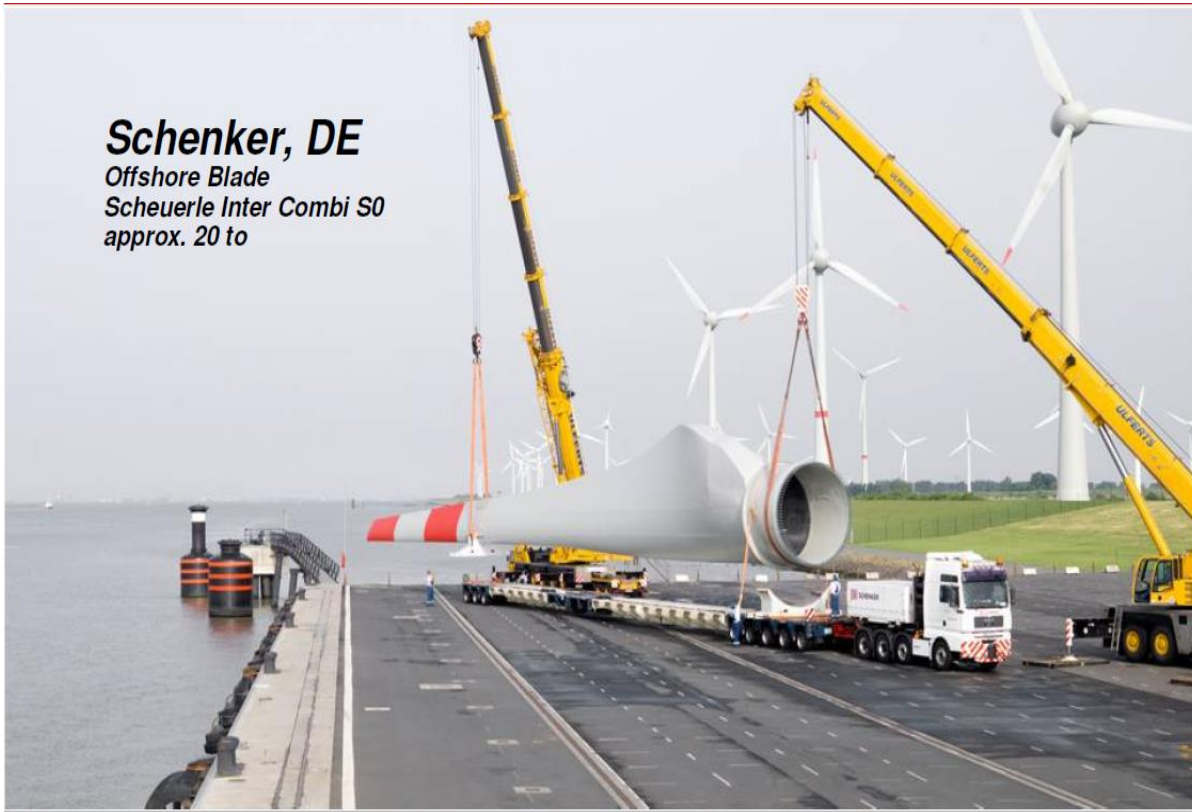
Figure 9 Blade being lifted onto SPMT.
