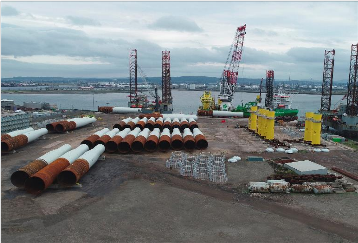
Figure 6: Monopiles, Transition Pieces and Anodes in typical storage at ASP
